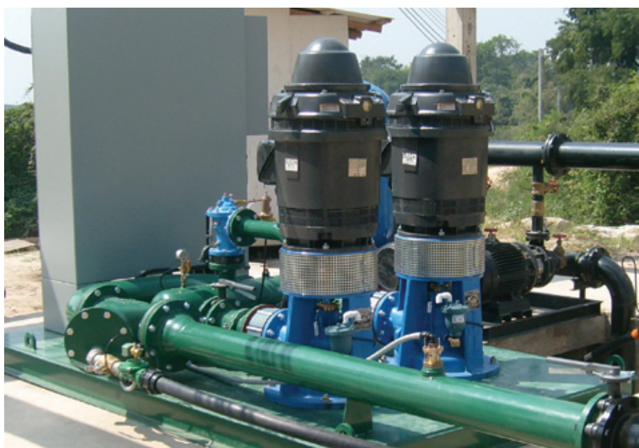
An installed Rain Bird Twin Vertical Turbine Pump Station complete with an optional Wye strainer.
