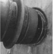
3. Place the Century-Line® Sleeve on the end cap. The sleeve should be cut 1/2" shorter than the width of the wall. Cut with a hand or power saw.
