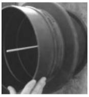
Place the sleeve over the end cap nailed to the form.
