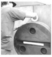
**7.** Wrap each seam with one wrap of 2" wide tape to bridge any possible gaps. **Note:** Tape not included.
