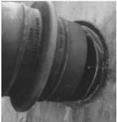
3. Place the Century-Line® Sleeve on the end cap. The sleeve should be cut 1/2" shorter than the width of the wall. Cut with a hand or power saw. Note: To insure minimum water migration, center the water stop in wall by cutting equal lengths from each end of the sleeve, except as noted below.
