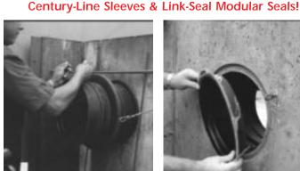
5. For additional stability, it's necessary to secure the sleeve with wire to the rebar. Insert the other end cap firmly and check that second end cap is positioned correctly and close the form.
