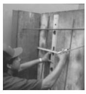
1. Measure the center line to position Century-Line® Sleeve end cap.
