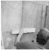
**2.** A 2x4 wood nailer is included. Fasten it along with the threaded rod directly to the concrete form. This provides support and helps center the complete Cell-Cast® disk assembly.
