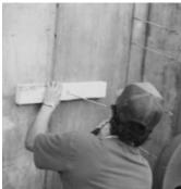
2. A 2x4 wood nailer is included. Fasten it along with the threaded rod directly to the concrete form. This provides support and helps center the complete Cell-Cast<sup>®</sup> disk assembly.
