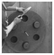
**4.** Secure the edges of the cell to the form using the provided steel spikes.
