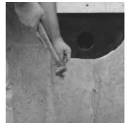
**9.** Chip excess concrete from the edge of the Cell-Cast<sup>®</sup> disk assembly and wall.
