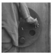
**3.** Slide the first Cell-Cast<sup>®</sup> disk over the threaded rod.
