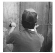
**1.** Locate center line where the hole is desired. This location will be used as a guide for the threaded centering assist rod.
