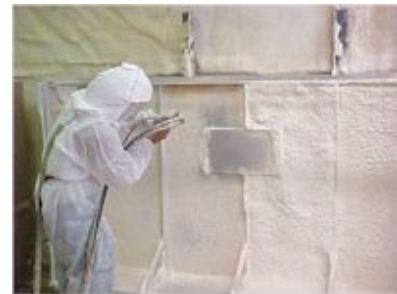
Spraying the Polyisocyanurate
