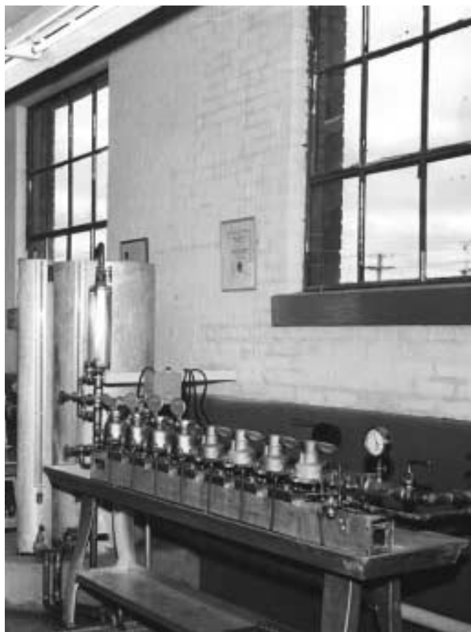
Testing 12 meters in series on an Indianapolis Type Test Bench. Electric control closes the valves at completion of test.
