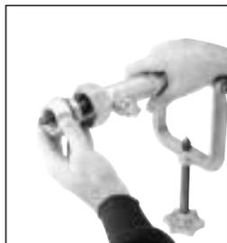
5. Mount the pipe saddle and corporation stop on the water main and tighten the saddle straps. Mount the Drilling Machine onto the corporation stop. **Check to be sure the corporation stop is fully open.**
