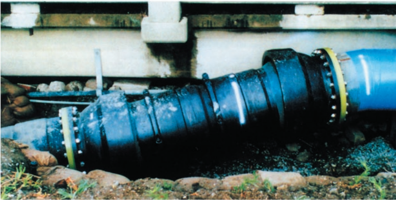
▲ Double-ball bridge crossing - 24" flange x flange with 16" expansion ▼ Double-ball tank connection - 6" flange x flange with 4" expansion
