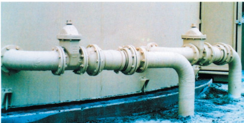
▲ Double-ball bridge crossing - 24" flange x flange with 16" expansion ▼ Double-ball tank connection - 6" flange x flange with 4" expansion
