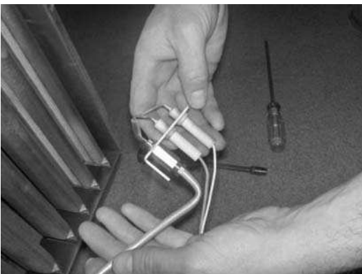
Step 17: Pilot removal for servicing.
