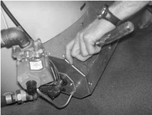
Step 1: Remove burner box cover screws
