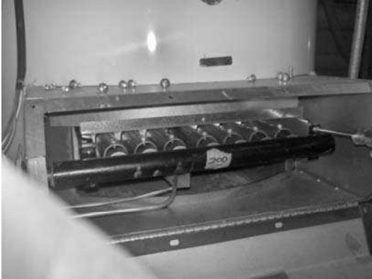
Step 7: Remove manifold bracket screws
