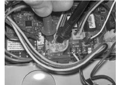
Checking MV & MV/PV control plug pins to gas valve for 24 volts output during heating cycle (pilot must be lit with no sparking).
