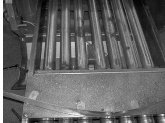
Step 14: Slide out burner assembly
