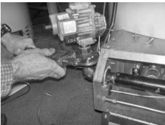
Step 5: Disconnect and Remove Gas Valve
