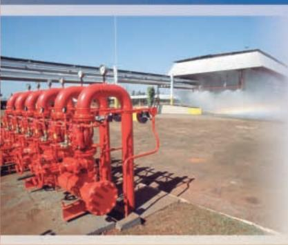
Bermad Deluge Valve is available in seven UL-LISTED Types, either electrically, hydraulically or pneumatically actuated, which can be utilized in various applications when provided with the appropriate operating system and accessories.
