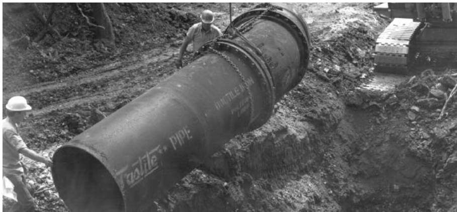
Installing a mechanical joint bend in a gravity sewer utilizing field-cut closure pieces to locate the fitting accurately.
