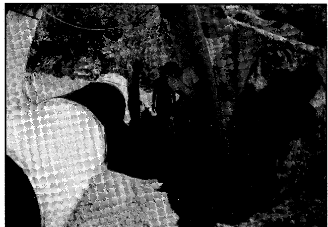
Figure 6. Soil being compacted around the pipe to be tested.
