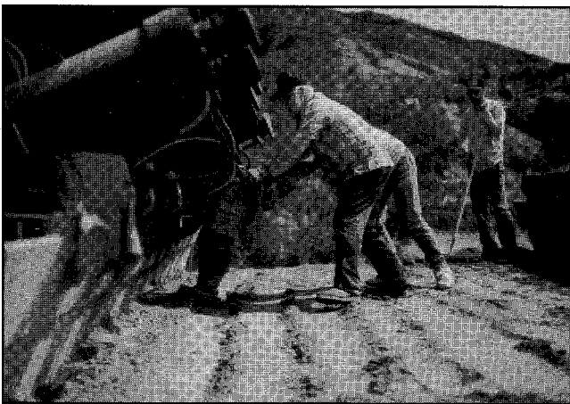
Figure 9. Soil being compacted as test cell filling is near completion.
